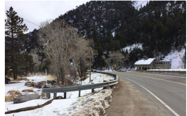
Site of culvert along CO 72 that will be replaced to meet current standards. (Photo: Estate Media)
